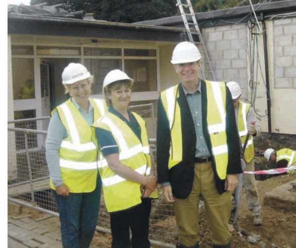
Inspecting redevelopment of Bishop's Castle Community Hospital
